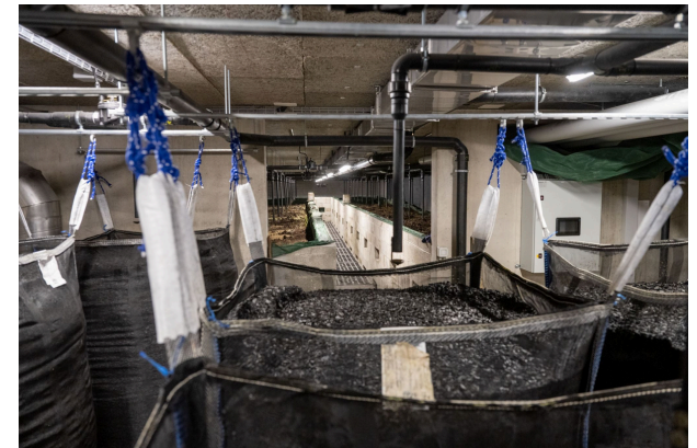
Photo: Circular sanitation installation, la Bistoquette
